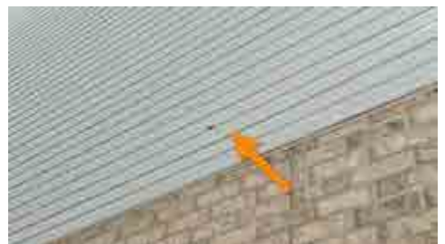
Damaged siding
